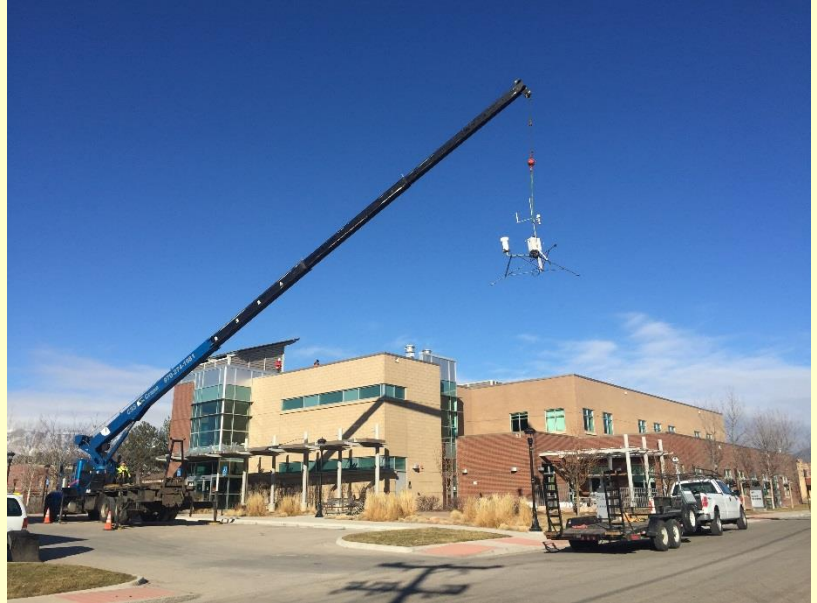
The meteorological and volatile organic compound equipment tripod is lifted onto the roof of the Rifle Library.
